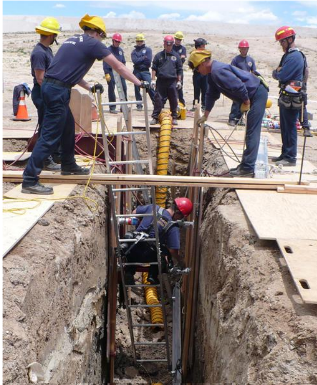
Figure 9-17 The safety officer should pick a good vantage point to see as much as possible. They also move around the rescue site periodically
