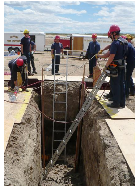
Figure 9-18 Place ladders for ingress and egress
